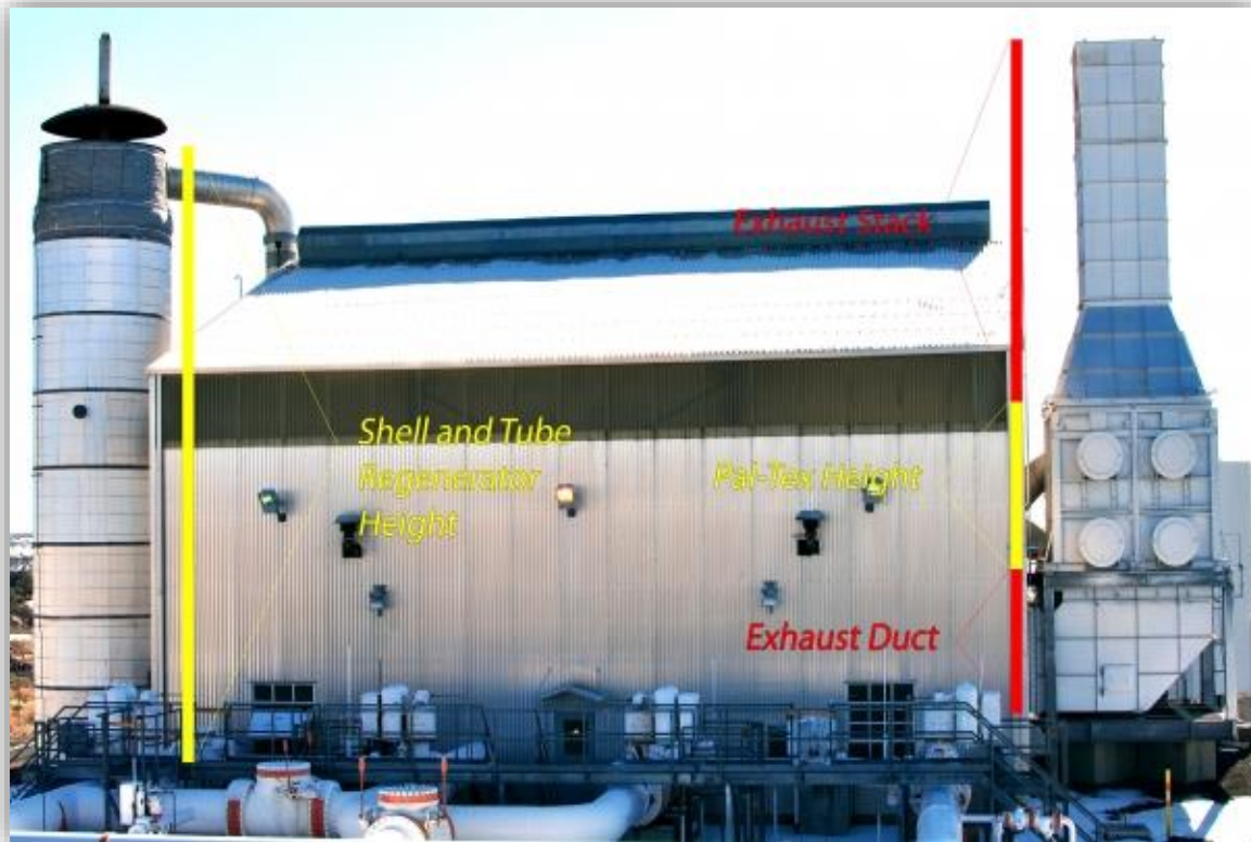
Fig : size comparison between PAL-TEX and another regenerator [1].
