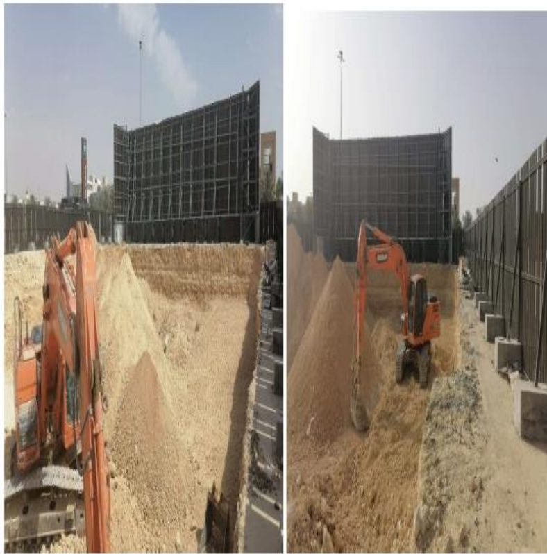
Excavation Work Progress
