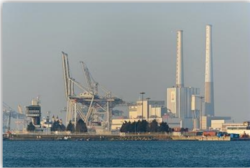
Figure 1-1: thermal power plant.
