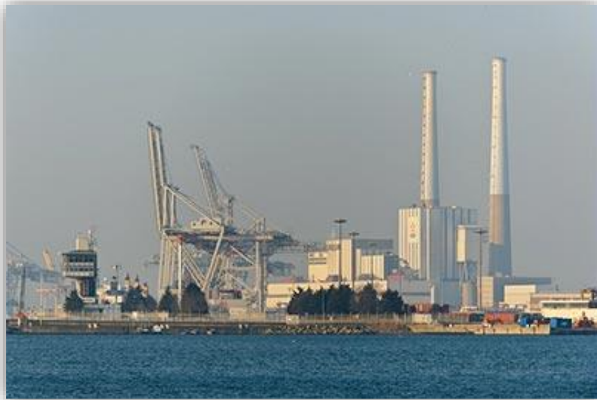
Figure 1-1: thermal power plant.
