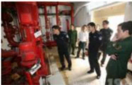
Firefighting facility issues
